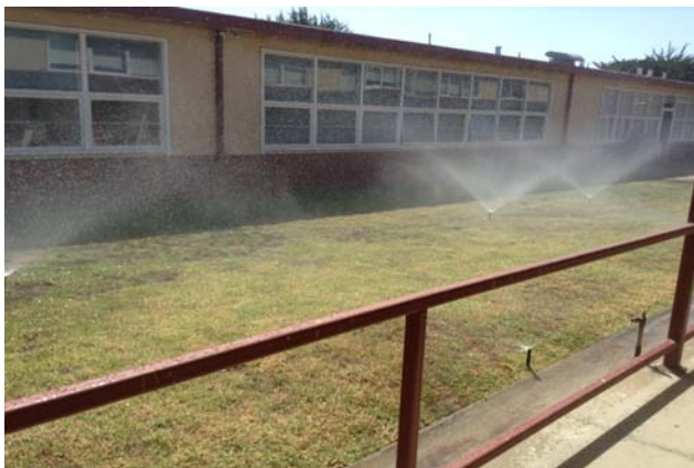
High Water-Use Inefficient Fixed Spray Sprinklers
